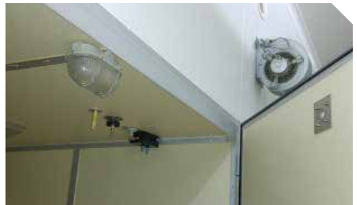
Figure 1 A hole drilled in the door and protected with a metal plate allows the insertion of the calibration probe close to the temperature sensor.
