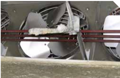
Figure 1 Blocked spray nozzles in setter No. 6
